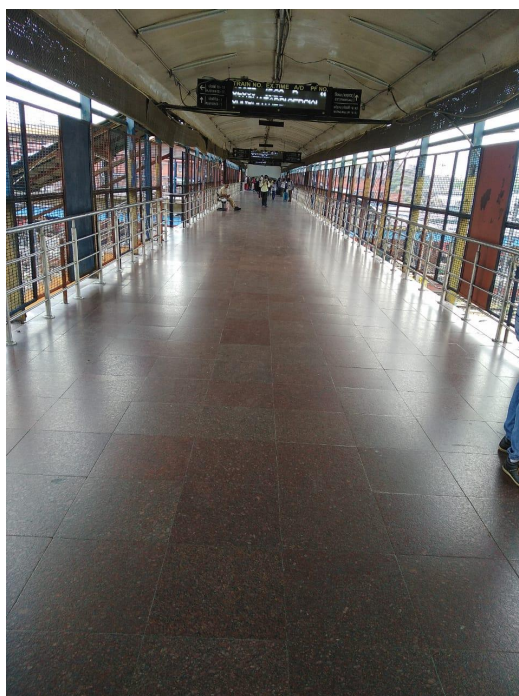
Fig 3. A Near Empty Foot over-bridge Source: First Author
