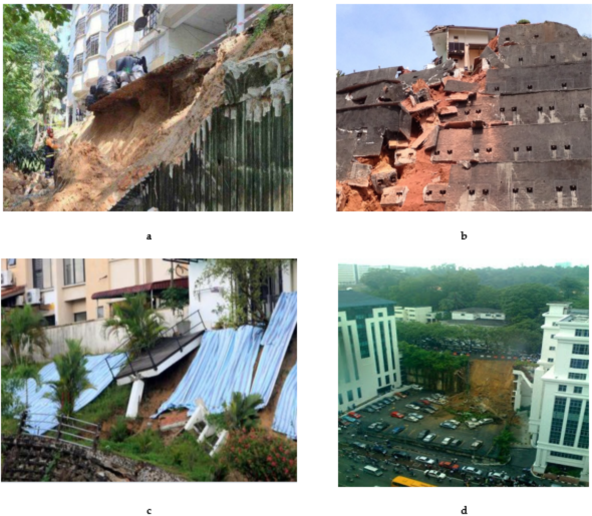
Fig 5. (a) Slope failures in Jalan Seri Penchala 1 in 2004, (b) Puncak Setiawangsa in 2011, (c) Taman Esplanad in 2006 and (d) Jalan Semantan in 2011
