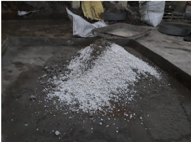
Figure 2. Dry mixed materials.
