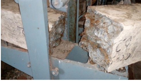
Figure 3. Hybrid fiber reinforced beam after flexural test.
