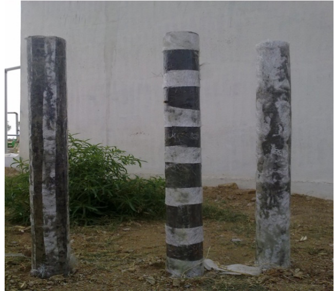
Figure 4. Column with FRP application.
