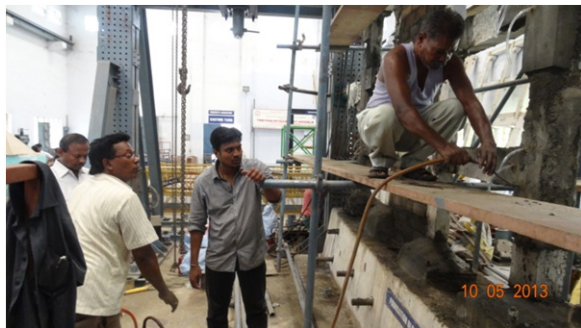
Figure 7. Grouting of retrofitted frame.
