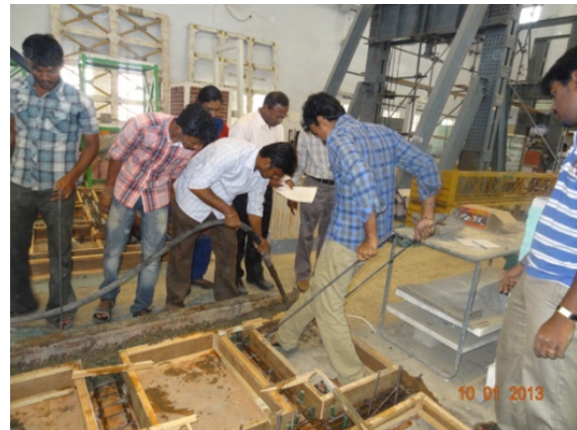
Figure 4. Placement of concrete.
