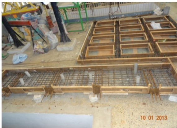
Figure 3. Wooden mould and reinforcement grill placed in position.
