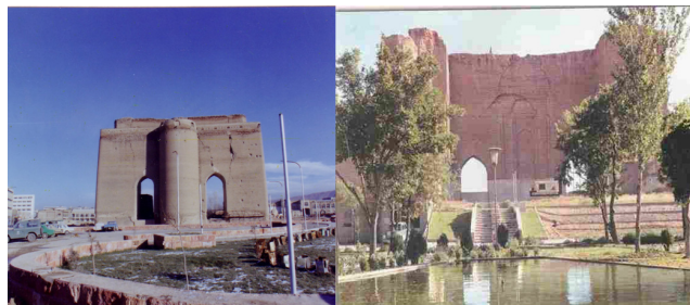
Figure 2. Southern façade of Arge- Tabriz ( right side), northern façade of Arge- Tabriz ( left side).
