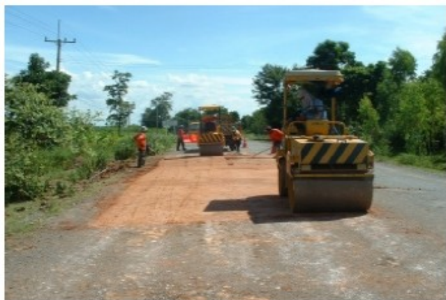
Fig.5. Pavement maintenance using lateritic soil cement
